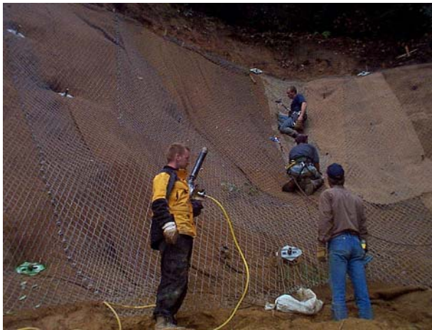
Fig. 10: Spike plate installation
