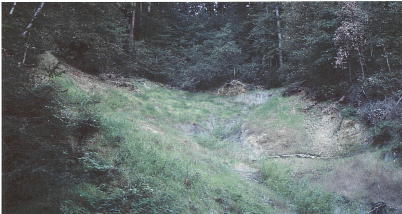
Fig. 12: Mesh is almost completely overgrown 16 months after installation.
