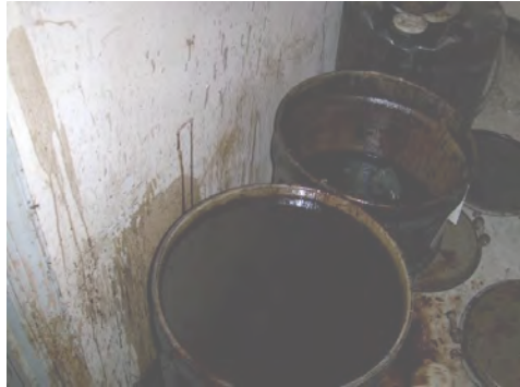
Poor solvent storage at a dry cleaning facility.
